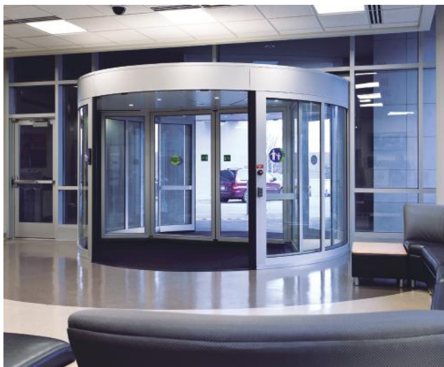
Foto: ASSA ABLOY Entrance Systems
