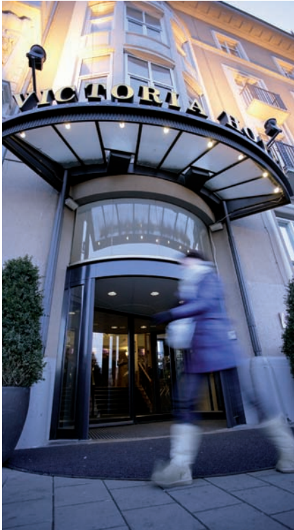
Foto: Assa Abloy Entrance Systems
